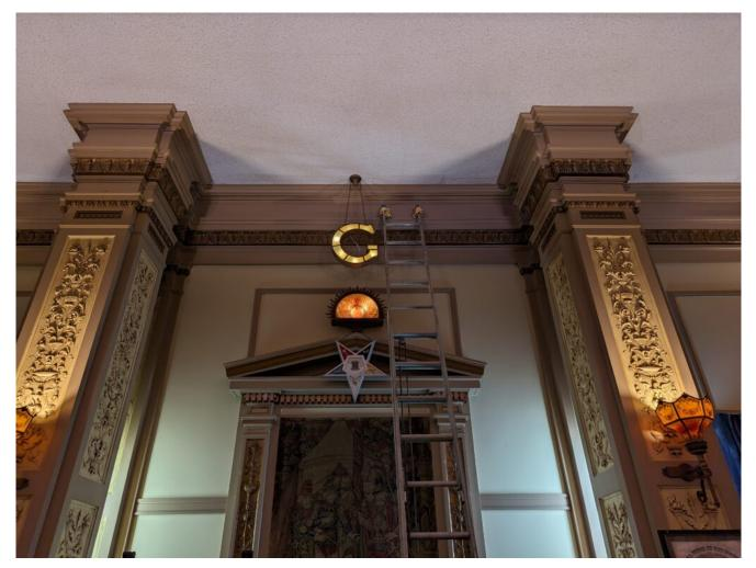
A couple of things to note about the G lamp. First, there is a single flathead screw on the back left side that holds the entire back piece in place. There is no hinge. Once that screw is removed, the entire back panel pulls off. Secondly, I was zapped twice when replacing the top dead center bulb. After replacing the back piece, I was able to touch the outer metal case without issue, but I think as some point the lamp will need to come down and be rebuilt so as not to zap any one else.
